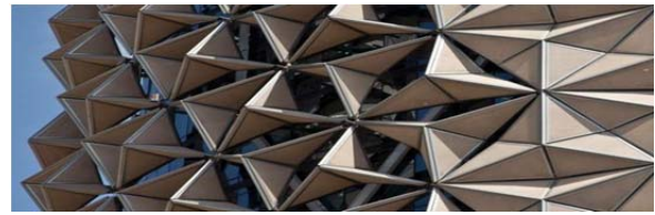
Fig. 6: L.R. Facade breathing foldable vents
